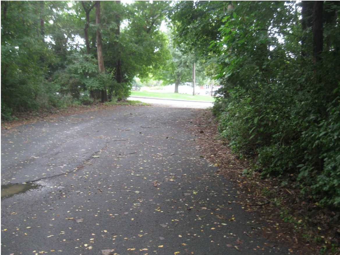
View of existing driveway looking toward Mill Road
