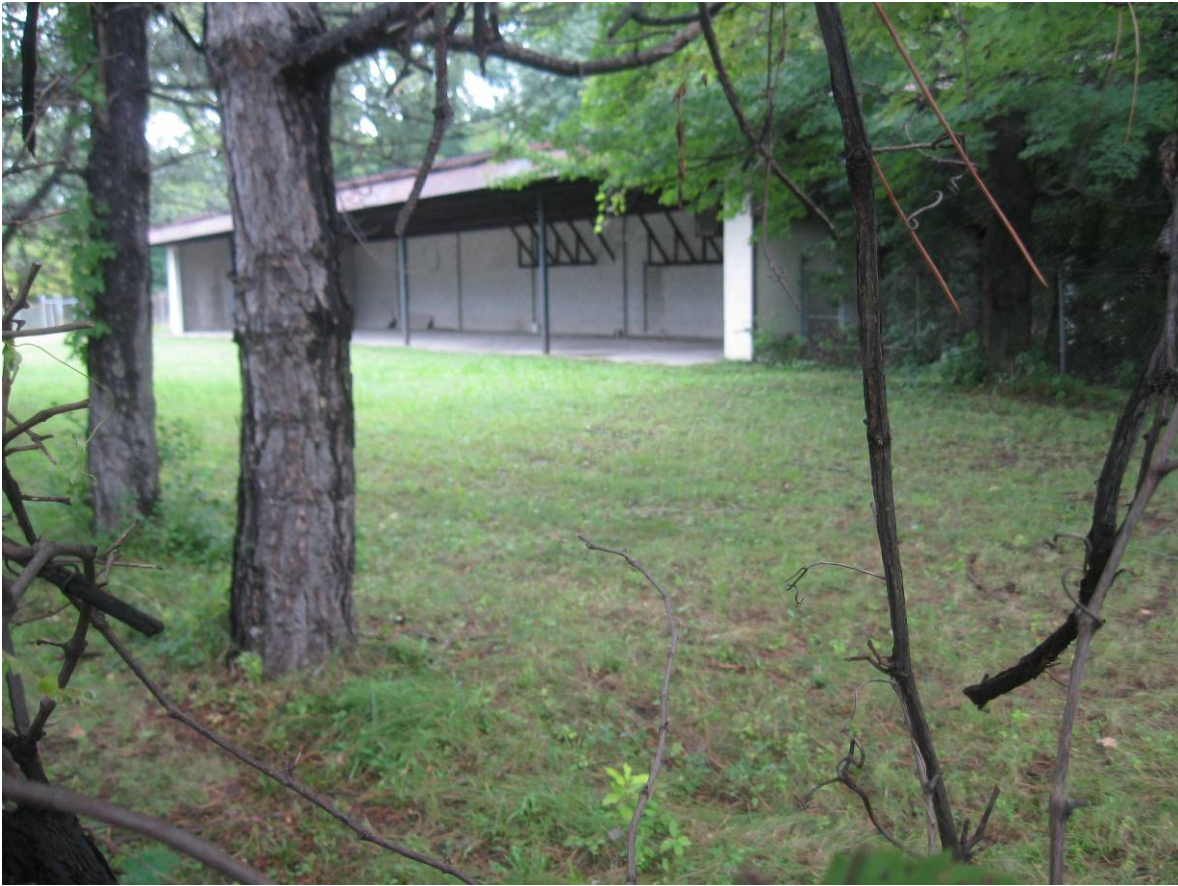
View of west side of main building
