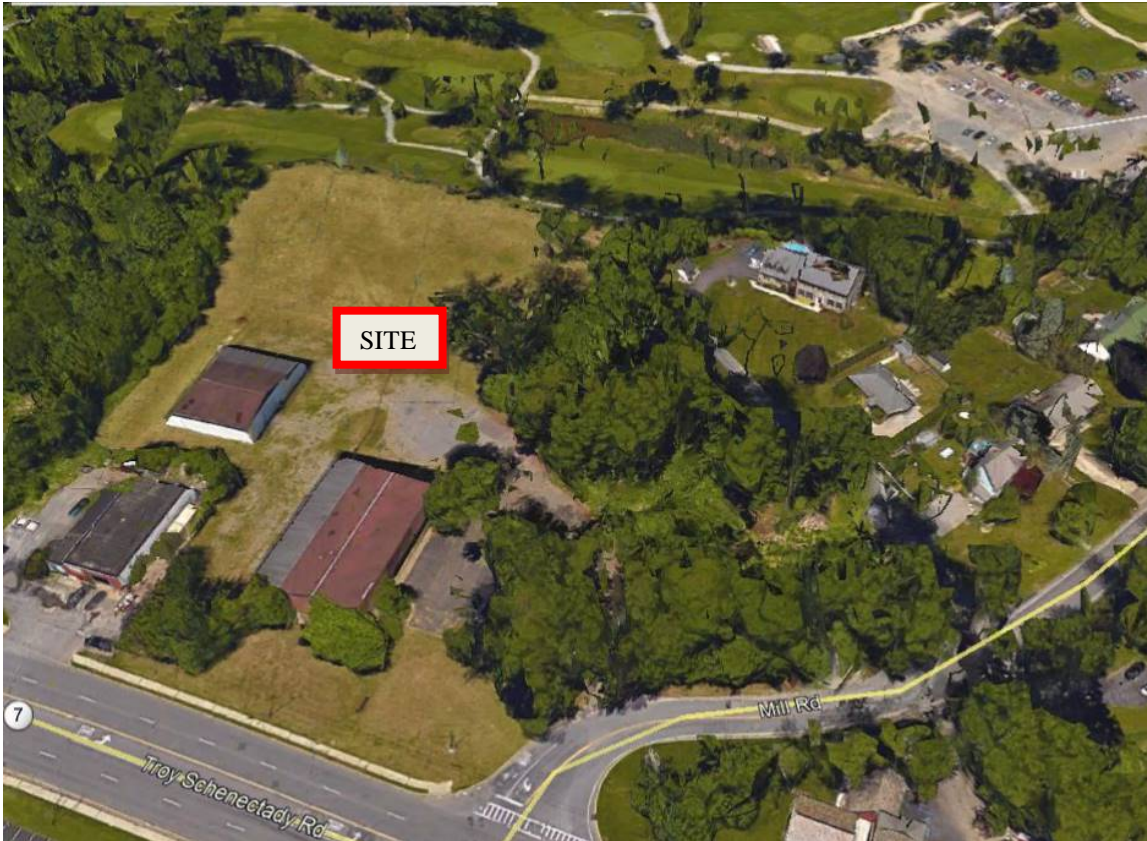
Fig. No. 1 - Aerial Photo of Existing Site
