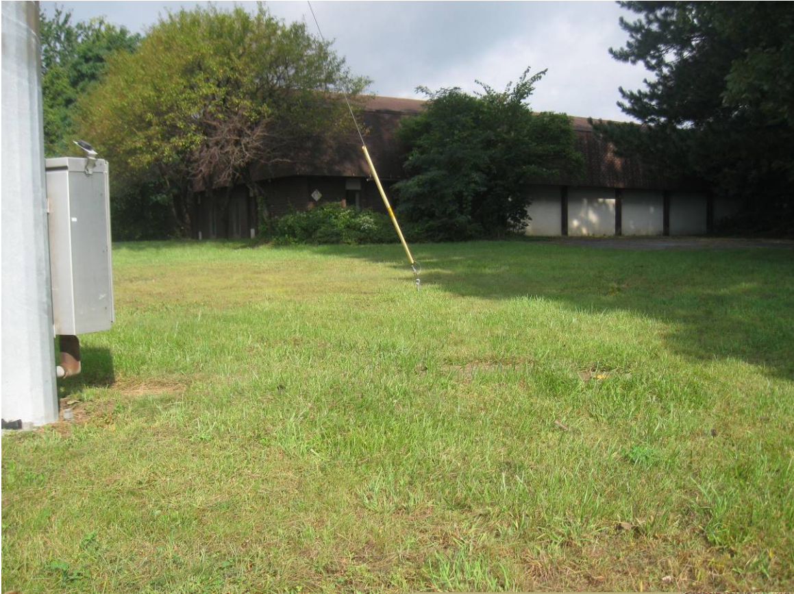
View of main building from Intersection of Troy-Schenectady Road and Mill Road
