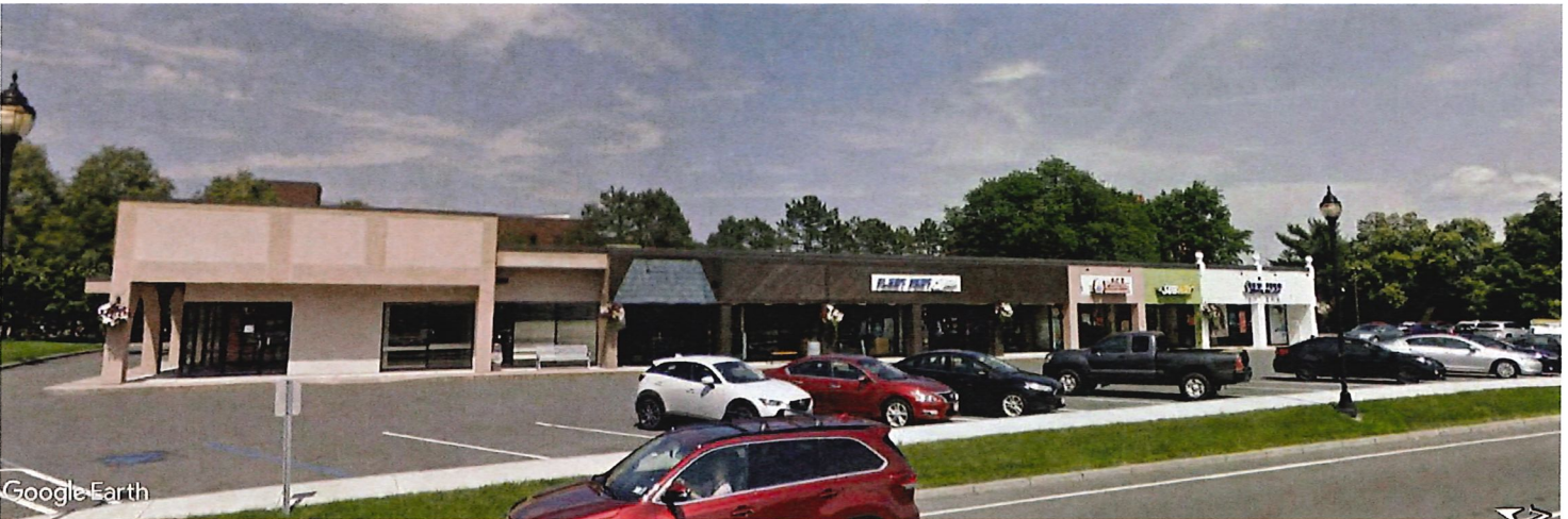
View of building from opposite side of Metro Park Road
