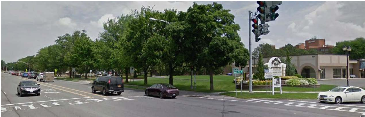
View from intersection of Wolf Road & Metro Park Road
